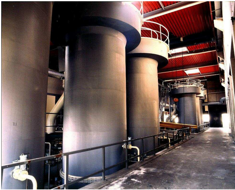
Figure 1. A full scale pellet reactors at the drinking water treatment plant "Weesperkarspel" of Waternet
