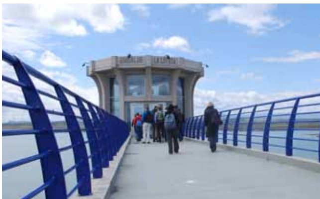
Inlet and outlet tower of the 'La Loteta' dam
