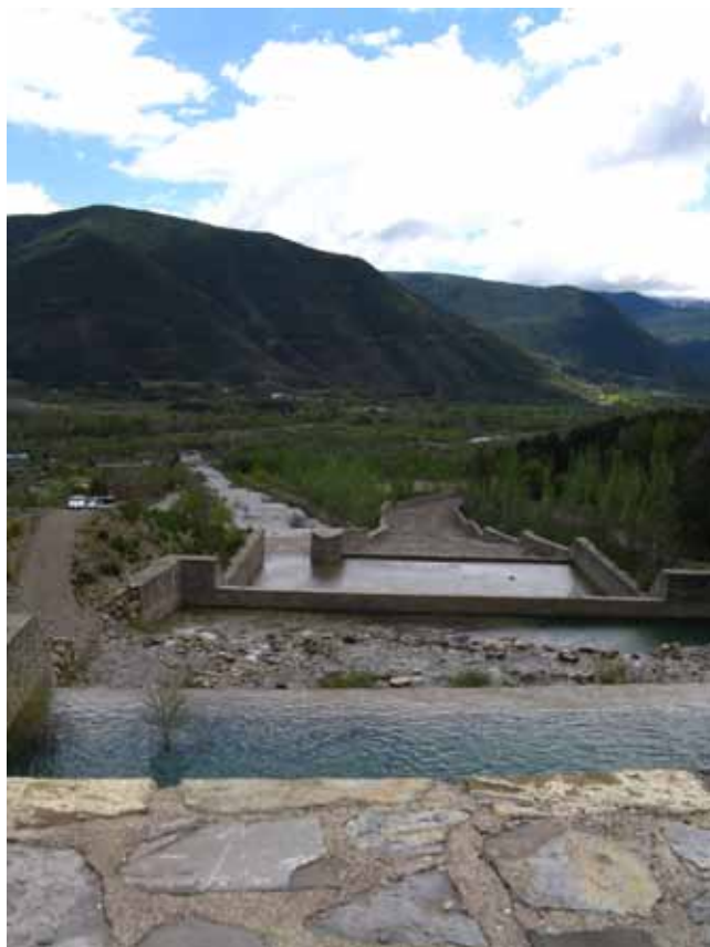
Normal riverbed to the left and emergency spillway at the right
