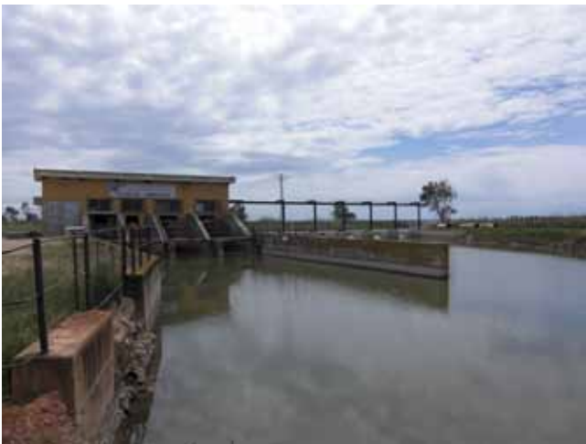
Figure 1: Archimedean screws. Water is brought from the irrigated fields to the sea.
