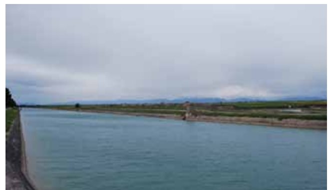
Large main irrigation canal (Canal de Monegros)
