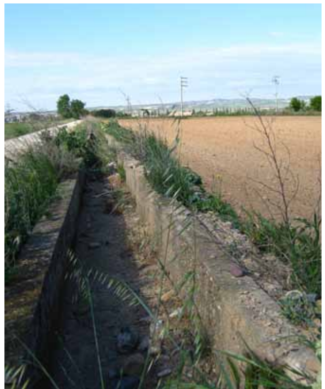
Small subordinate irrigation channel near Ontinar de Salz
